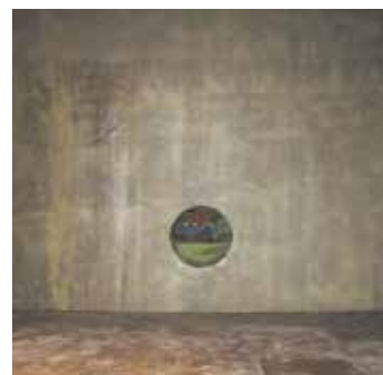
RC薬品貯蔵槽
